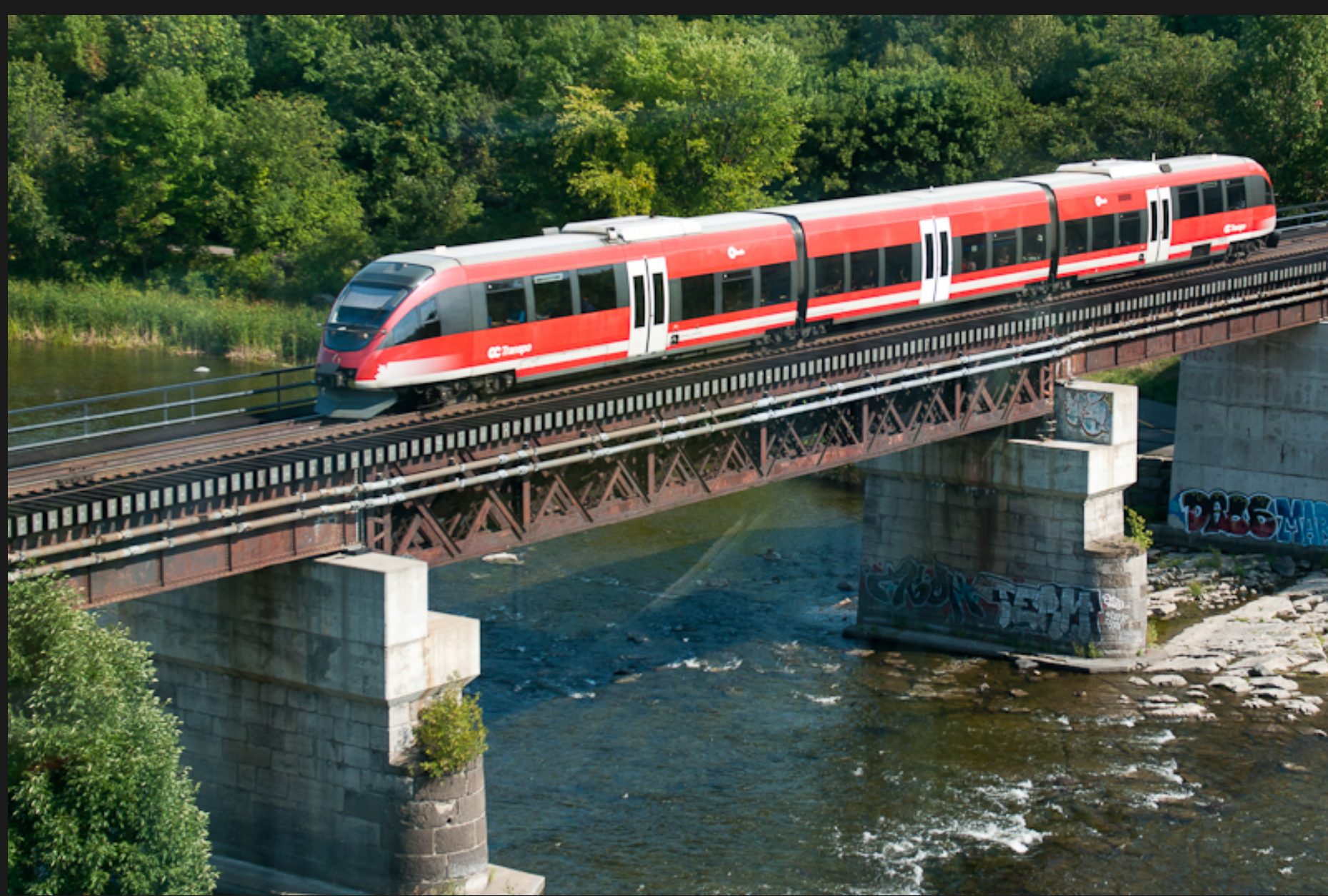
The O-Train will close for construction at the end of the school year in April. (Photo by Pedro Vasconcellos)
